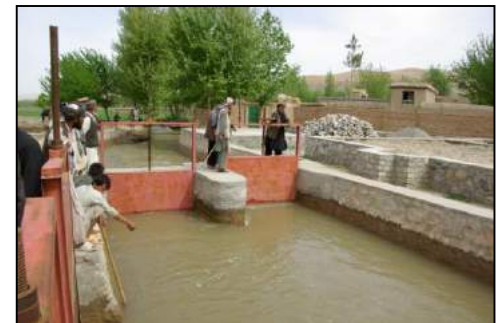
Rehabilitating an irrigation gate
