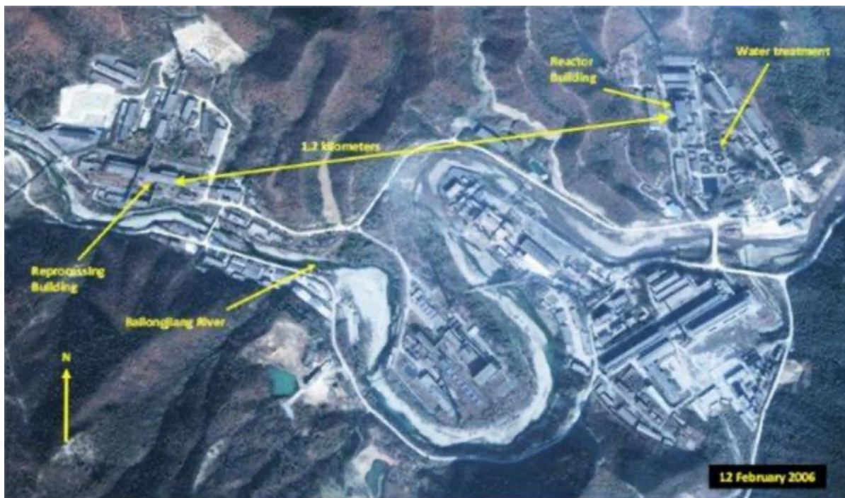
Figure 15. The reactor and reprocessing areas of the 812 Plant.
