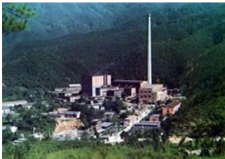
Figure 16. Ground view of the 812 Plant reactor area. 32
