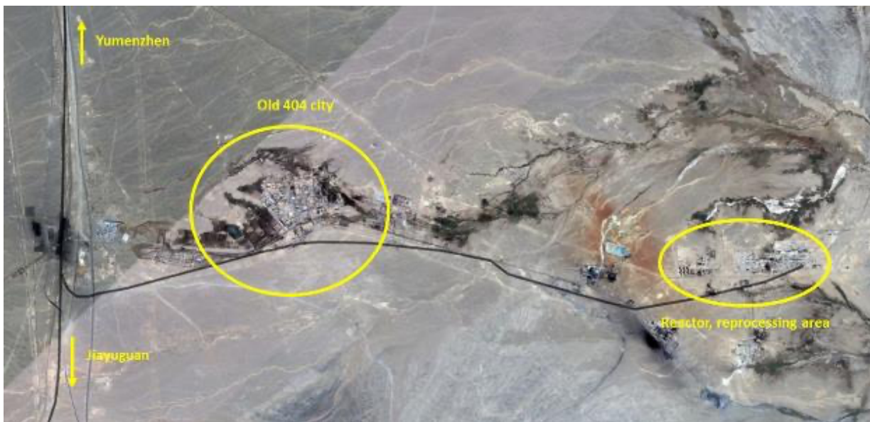
Figure 4. Overview of the 404 Plant site
